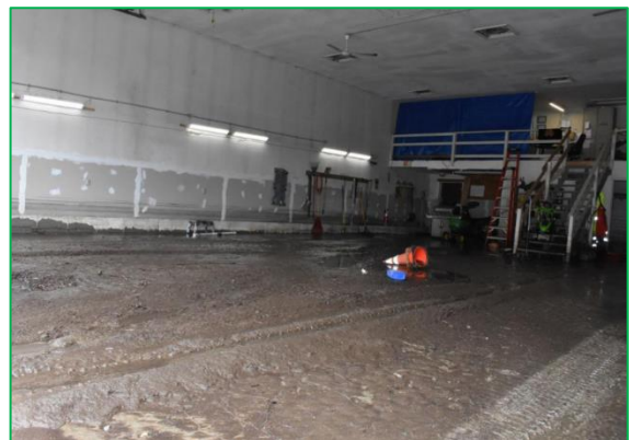
Town Garage, after July 2019 flood event Photo Credit: Bea Lewis, Union Leader
