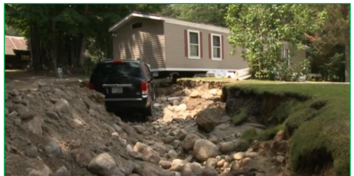
Damage to home on Sculptured Rocks Road, July 2019 Photo Credit: Snip from https://www.wmur.com/article/groton-homeowners-dealing-with-devastating-flood-damage/28391500
